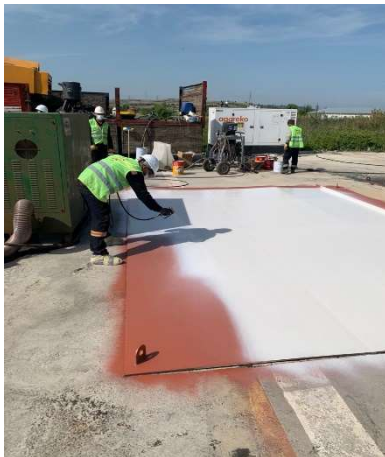
PUMMA application by airless sprayer.
