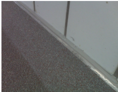
Completed cove with profile
